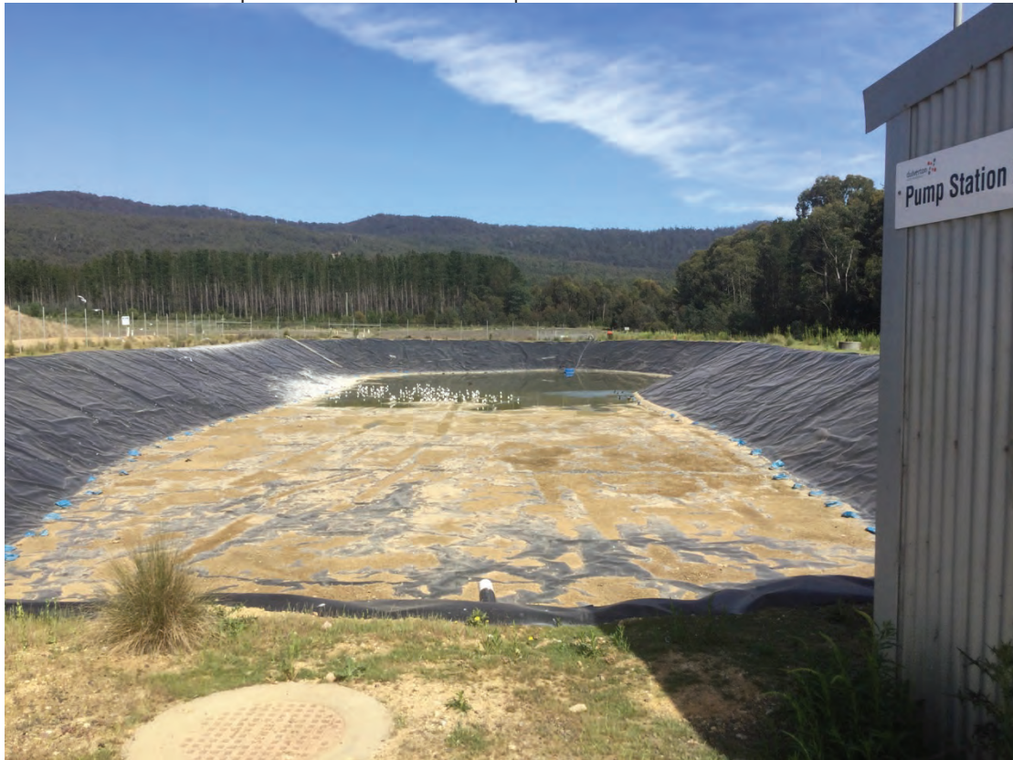
Photo below N° 4 = The leachate pond that was relined to give it extra capacity and remove sludge.
