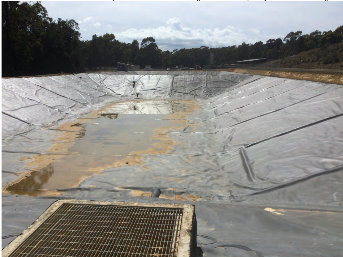
Photo below N° 4 = The leachate pond that was relined to give it extra capacity and remove sludge.
