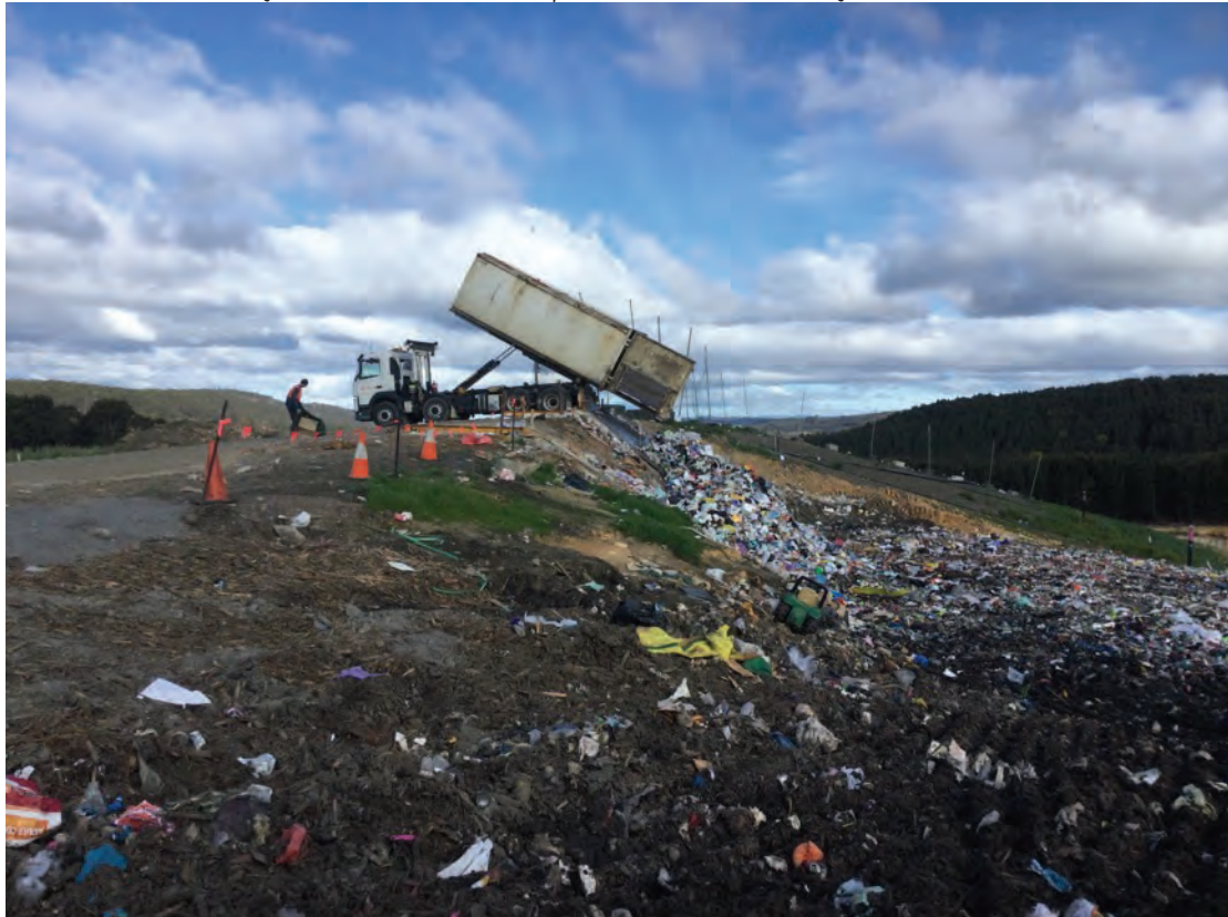
Photo below N° 2 = Recycle waste site needs compaction soon after delivery to control wind-blown litter.
