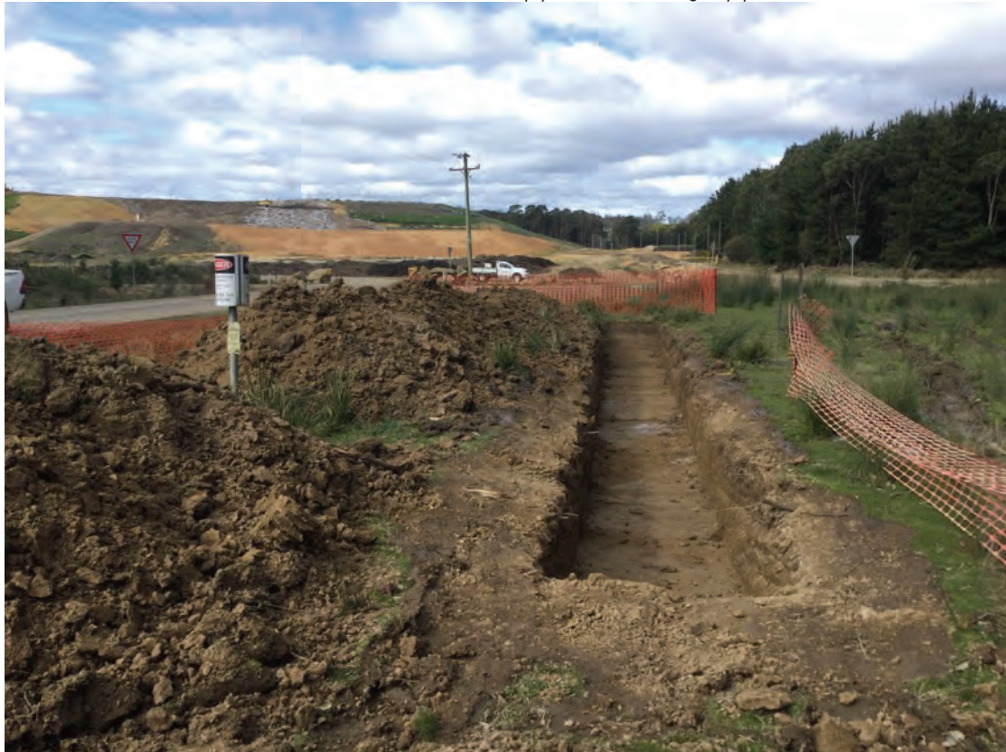
Photo below N° 4 = Test excavation ditch area for water pipe located near gas pipeline.
